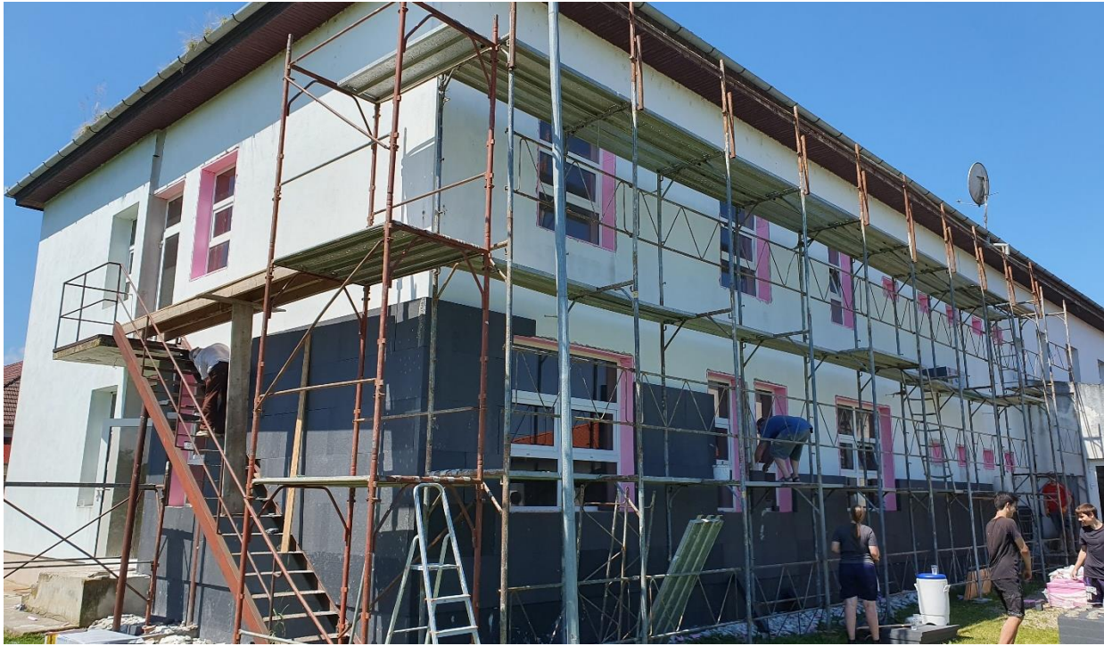
Adding insulation to the back of the Bible college building
